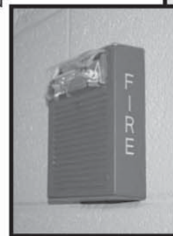
Fire Alarm Horn/Strobe
